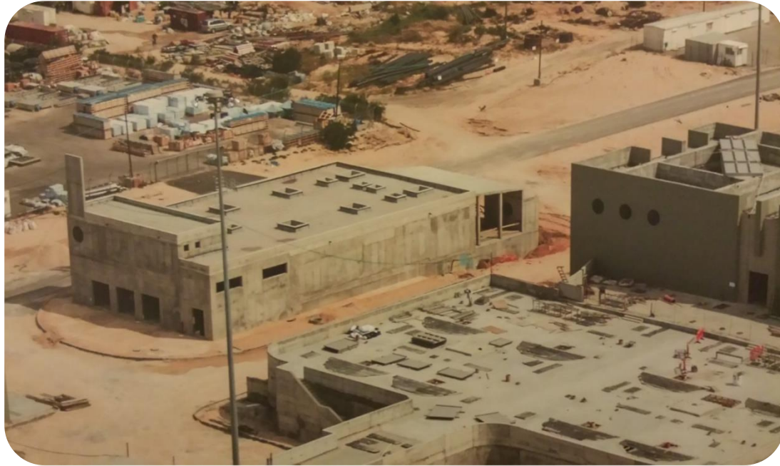
BTF + BF Concrete Reactor
