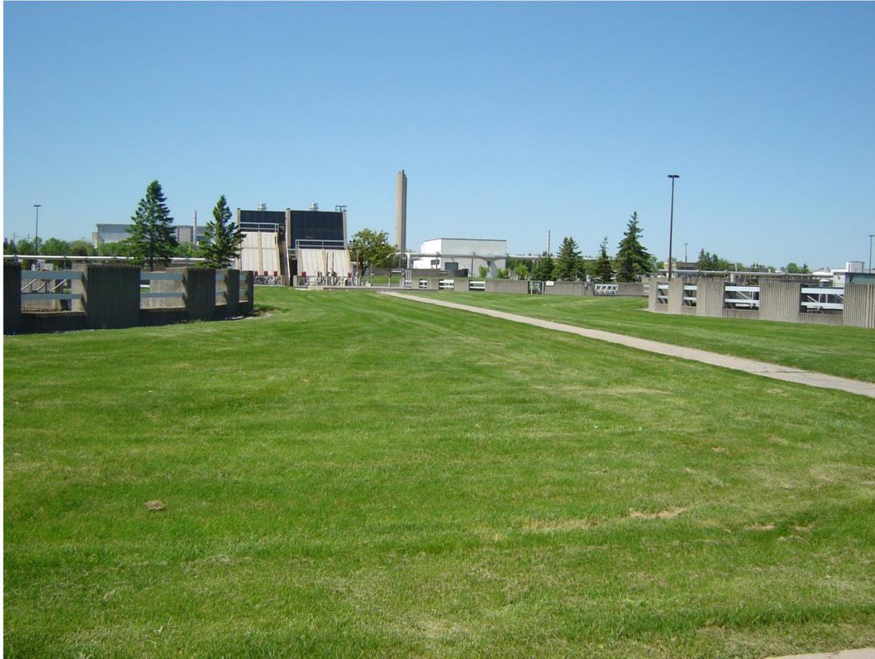
Duffin Creek Water Pollution Control Plant
